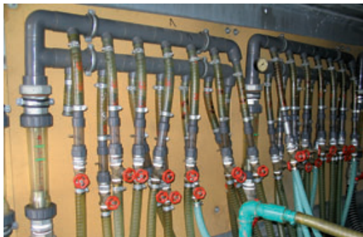
VAK 200 in use for 20 extraction wells
